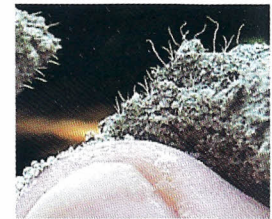
Or break open a thin piece of hard concrete
